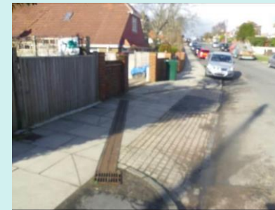
Figure 20 - Gullies and Slot drains on Warmdene Road [Available online ].
