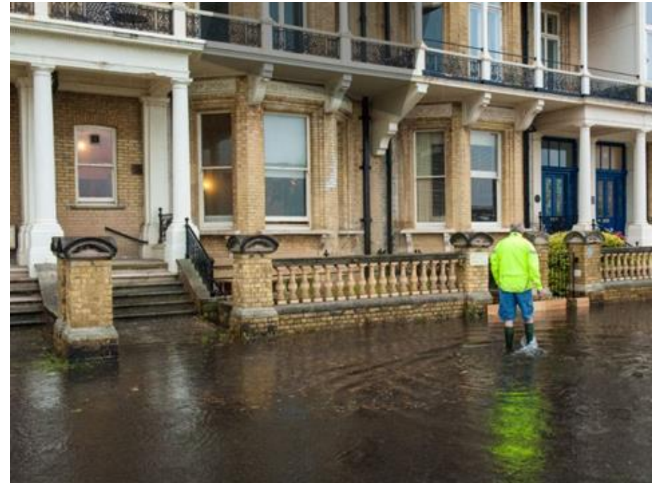
Figure 1 - Flooding in Brighton (Source: Brighton & Hove City Council, n.d. (online). Available at: brighton-hove.gov.uk ).
